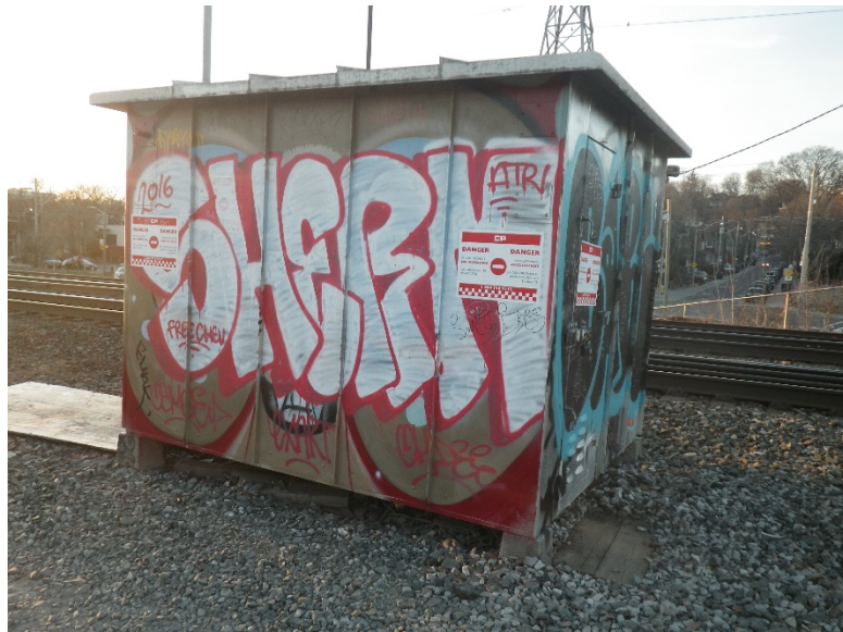
Figure 5. Red and white “No Trespassing” signs installed on the signal bungalow over red and white graffiti (Source: TSB)
