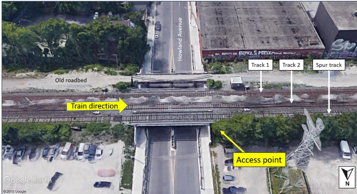
Figure 1. Howland Avenue grade-separated crossing where the teenagers accessed the right-of-way, looking south down Howland Avenue (Source: Google Earth, with TSB annotations)
