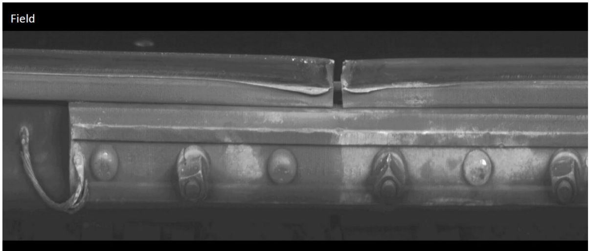
Figure 9. Field-side standard joint bar (Mile 197.4751) showing rail head end batter (Source: Canadian National Railway Company)
