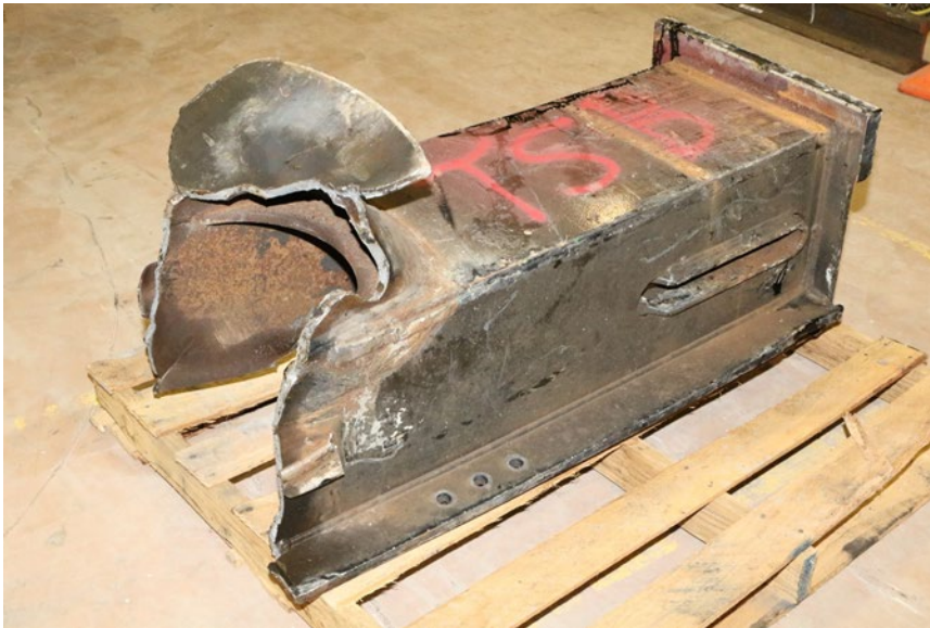
Figure 19. Stub sill, head brace and reinforcing pad (Source: TSB)
