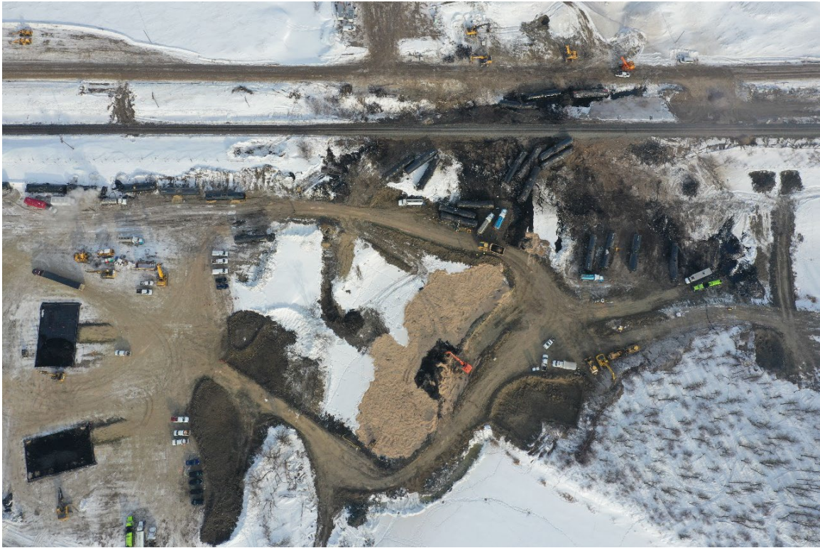
Figure 7. Aerial view of site remediation activities (Source: GHD)
