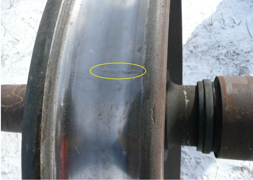
Figure 2. Impact mark on VMSX 280746 R4 wheel tread (Source: TSB)
