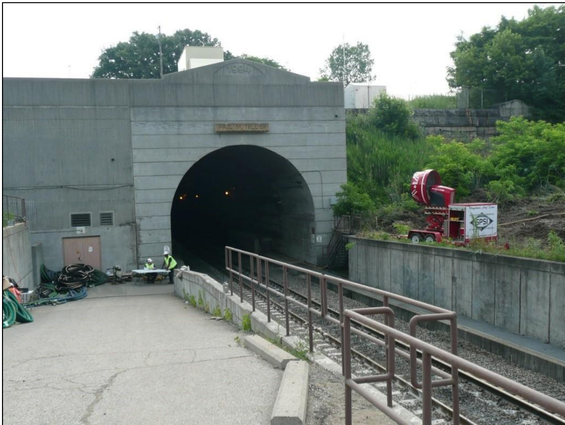
Figure 2. Port Huron tunnel portal in the United States (Source: TSB)
