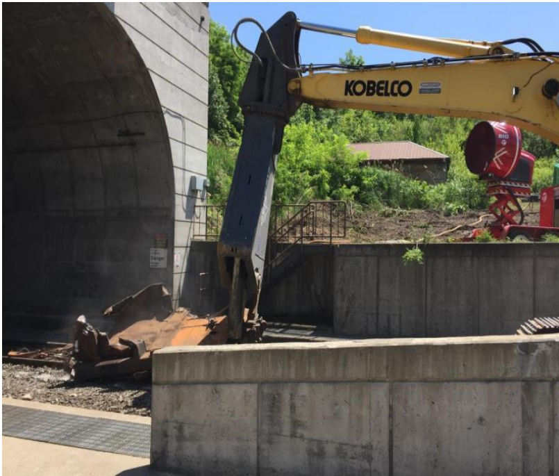
Figure 14. Car DJJX 30478 A-end shear plate and stub sill were removed from the tunnel (Source: Environmental Protection Agency)
