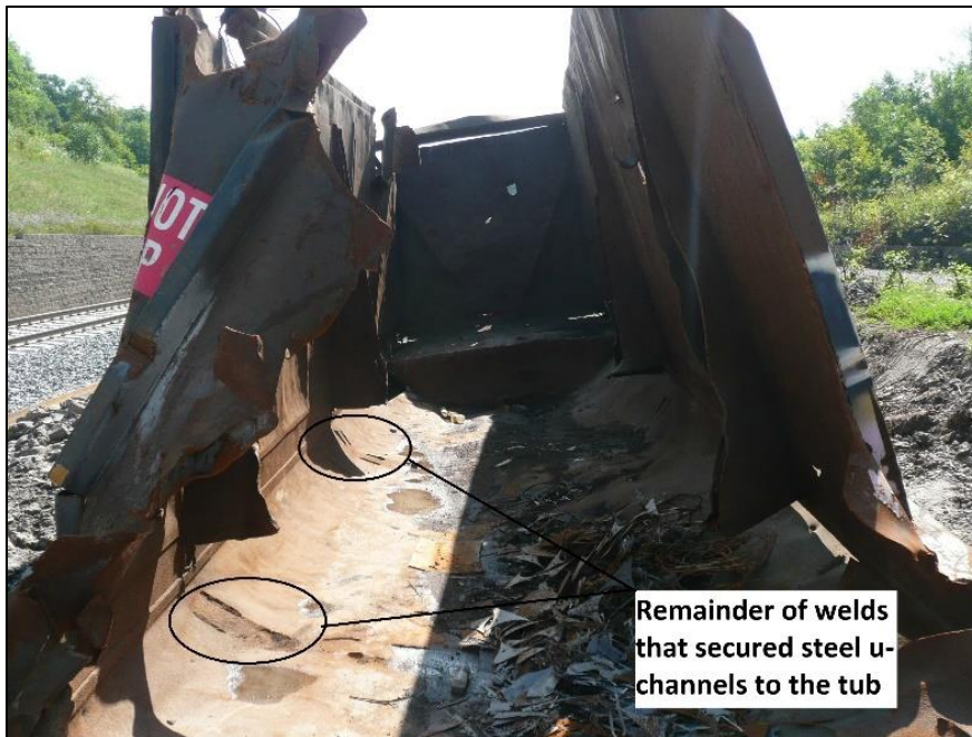
Figure 26. Car DJJX 30478, view inside the car from the A-end (Source: TSB)
