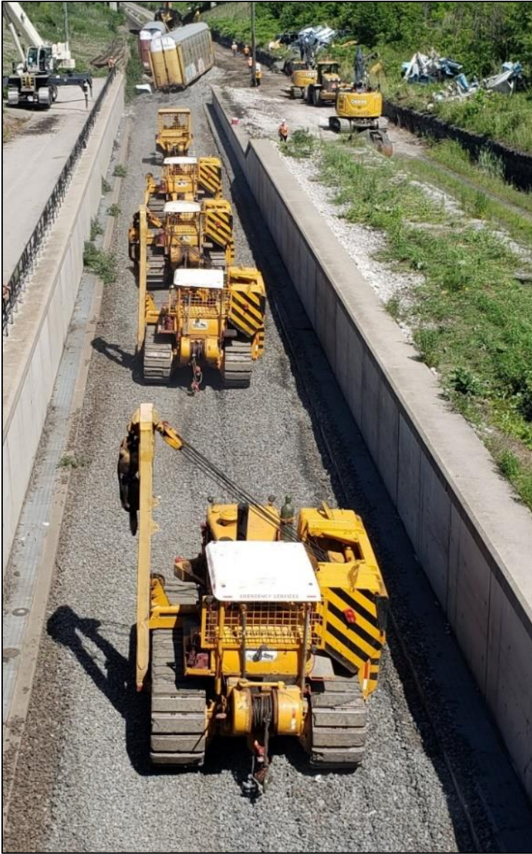
Figure 18. Heavy equipment used in clearing activities (Source: TSB)
