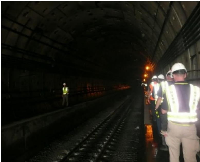
Figure 5. Tunnel entry from the U.S. side (Source: TSB)
