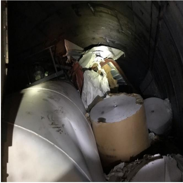
Figure 10. Example of derailed cars and lading blocking the tunnel on the U.S. side (Source: Federal Railroad Administration)
