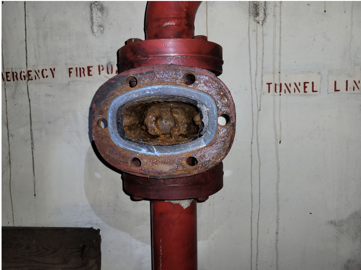
Figure 21. The isolation valve, showing the disconnected gate (Source: TSB)
