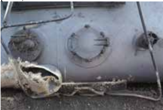
(e) Top fittings, manway and PRD
