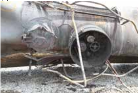
(e) Manway and top fittings
