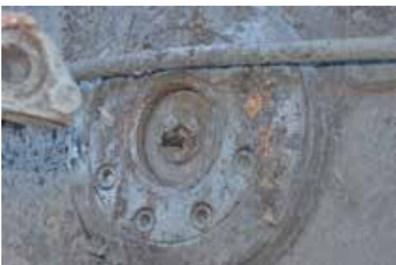
(g) BOV (RSI-AAR Safety Project photo)
