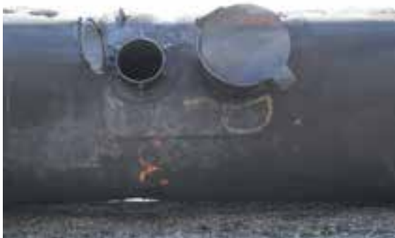
(g) Top fittings and manway
