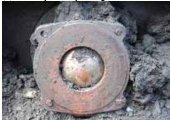
(f) Close-up showing partially open BOV ball
