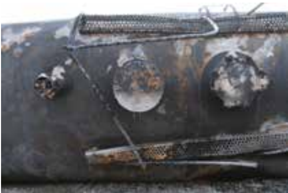
(g) PRD, top fittings and manway
