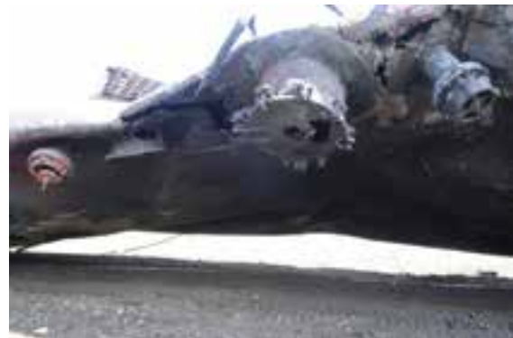
(h) Top fittings, manway and PRDs
