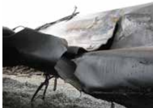
(h) Rupture in shell between BOV and B end
