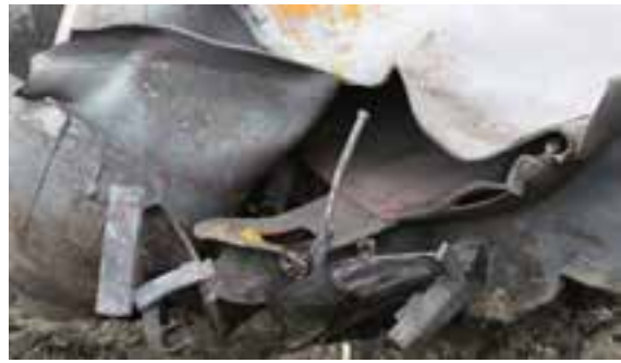
(b) Close-up showing separations at B end stub sill and BR body bolster
