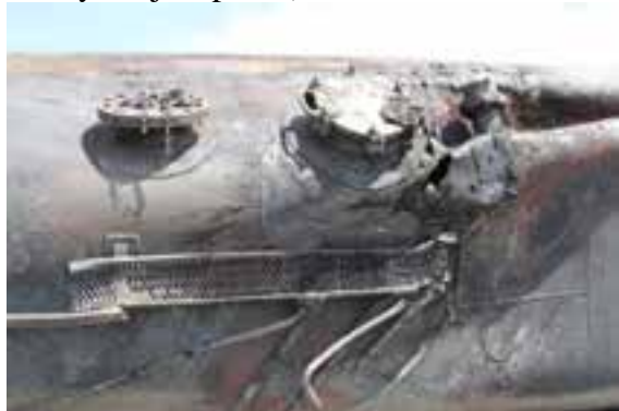
(f) Top fittings, manway and PRD
