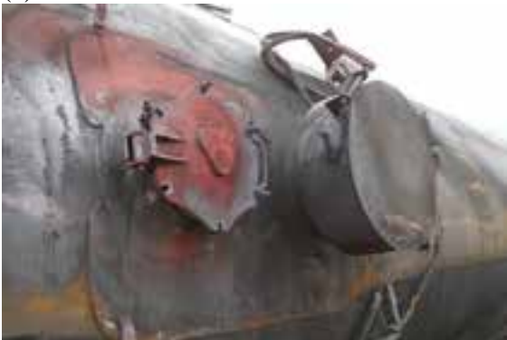
(g) Top fittings and manway
