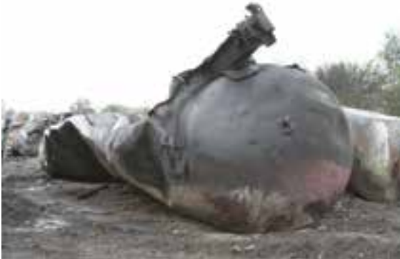
(c) Shell viewed from the A end
