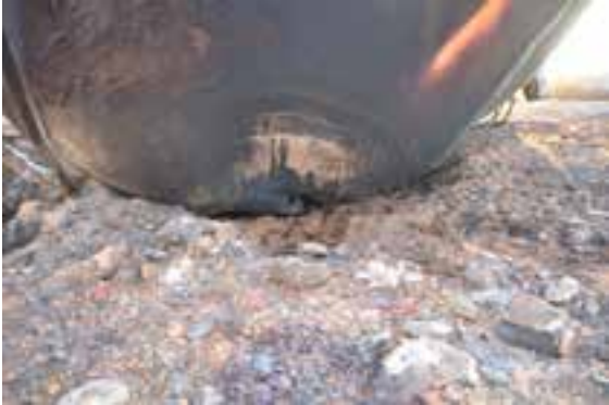
(c) In-situ photo showing small puncture at the left edge of the A end (RSI-AAR Safety Project photo)
