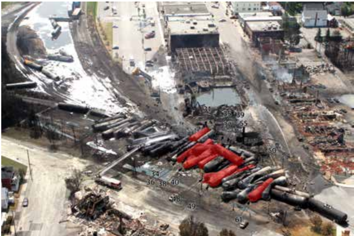
Figure 11: Aerial photograph showing cars with burn-throughs indicated in red
