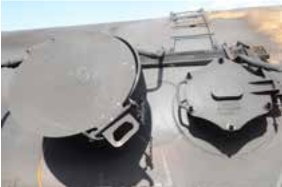
(g) Top fittings and manway
