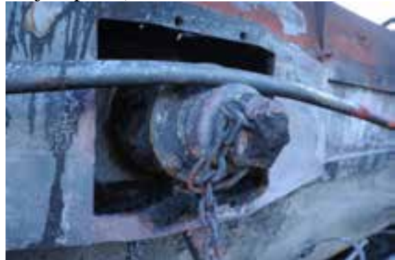
(f) Close-up showing product residue on BOV
