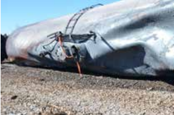
(c) Shell (RSI-AAR Safety Project photo)
