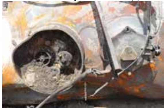
(f) Top fittings and manway
