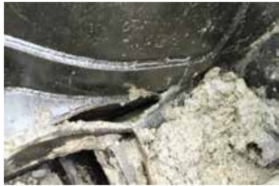
(b) Close-up showing failed B end stub sill welds
