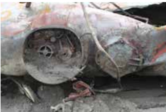
(g) Top fittings and manway
