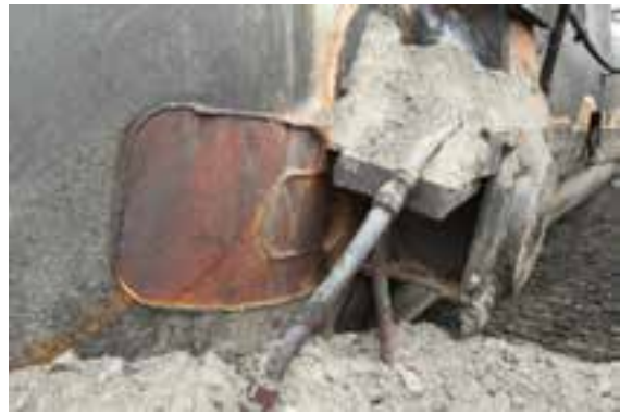
b) Close-up showing broken B end stub sill
