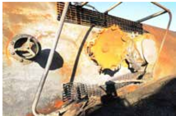
(f) PRD, manway and top fittings
