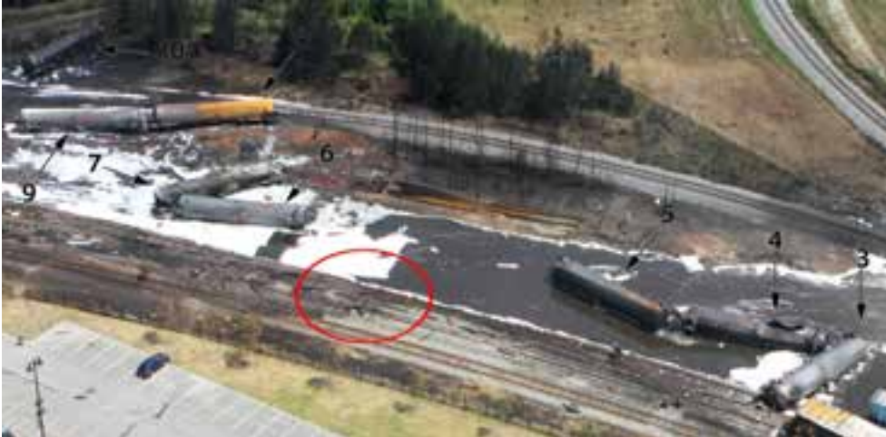
(a) Aerial view looking north showing consist no.3 through 10. The broken portions of yard tracks 1 and 2 are circled.
