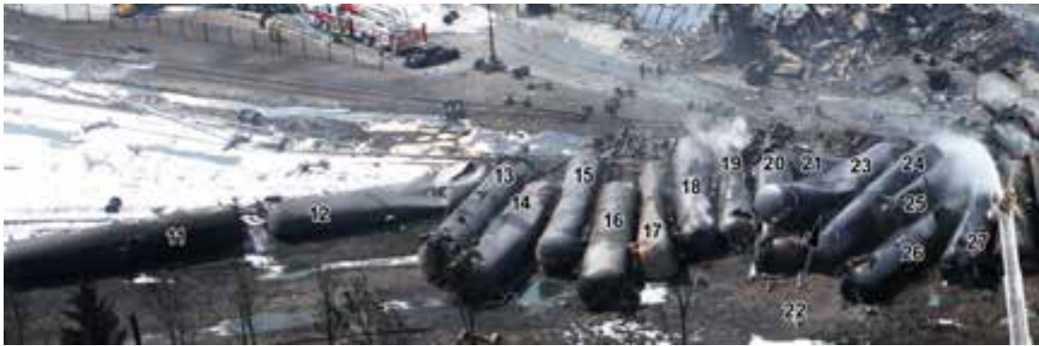
(a) View looking south
