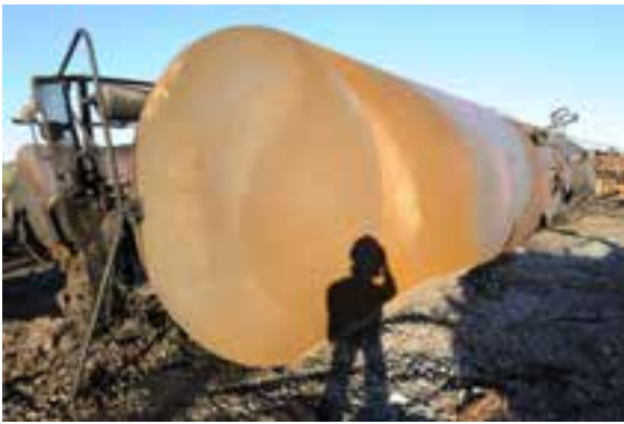
(a) Shell top viewed from the B end
