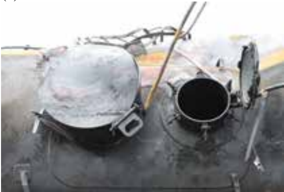
(e) Top fittings and manway
