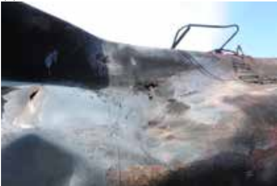
(e) Close up of shell puncture and burn-through
