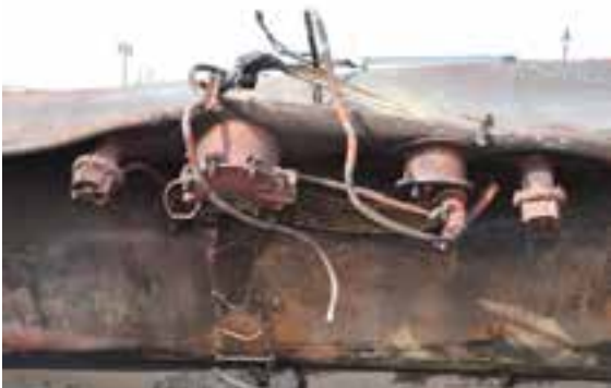
(g) Manway and top fittings (RSI-AAR Safety Project photo)
