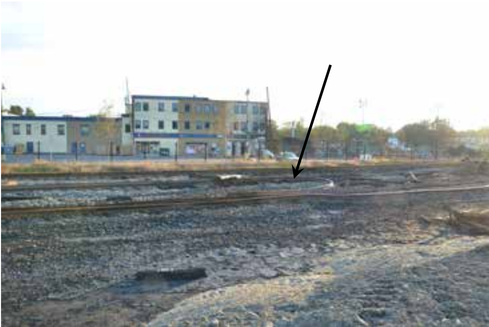
(d) In-situ photo showing a close-up of the area circled in Figure B-3a. The arrow points to a broken rail bent back 180 degrees (RSI-AAR Safety Project photo).
