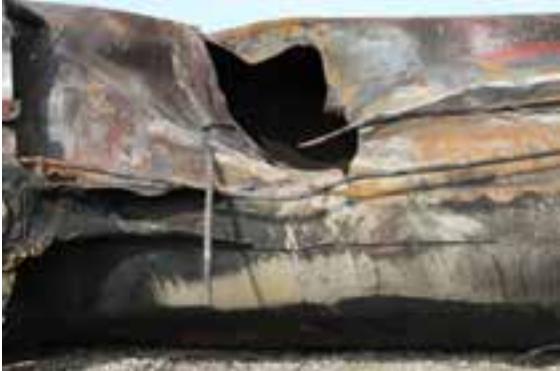
(e) Close-up of large puncture in the shell
