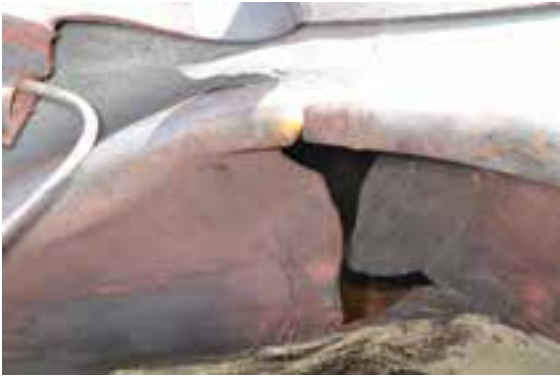
(c) Close-up showing a rupture in the area circled on (a) (RSI-AAR Safety Project photo)
