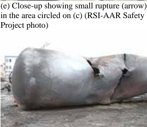
(g) Large ruptures in the shell
