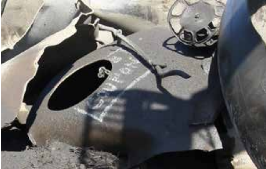
(a) Sheared-off head with a round hole where the coupon has been cut out using water-jet equipment.
