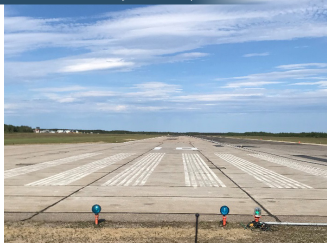
PHOTO 4. Runway under repair
