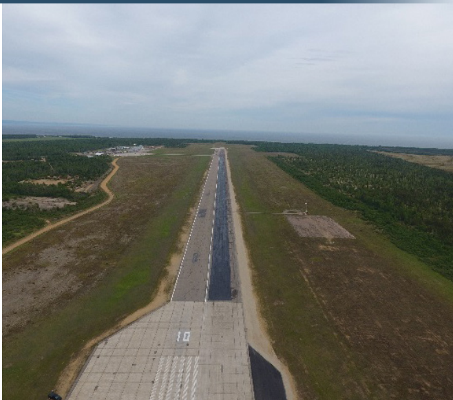
PHOTO 1. Airport undergoing runway repairs
