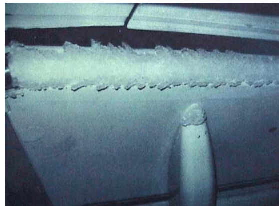
Photo 1. Ice accretion on main flaps leading edges from a December 1998 A321 event
