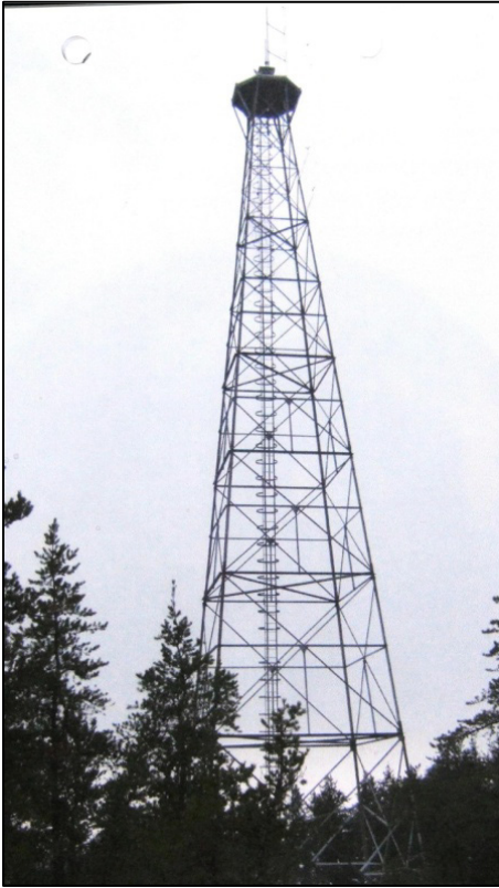
Photo 1. The tower prior to impact
