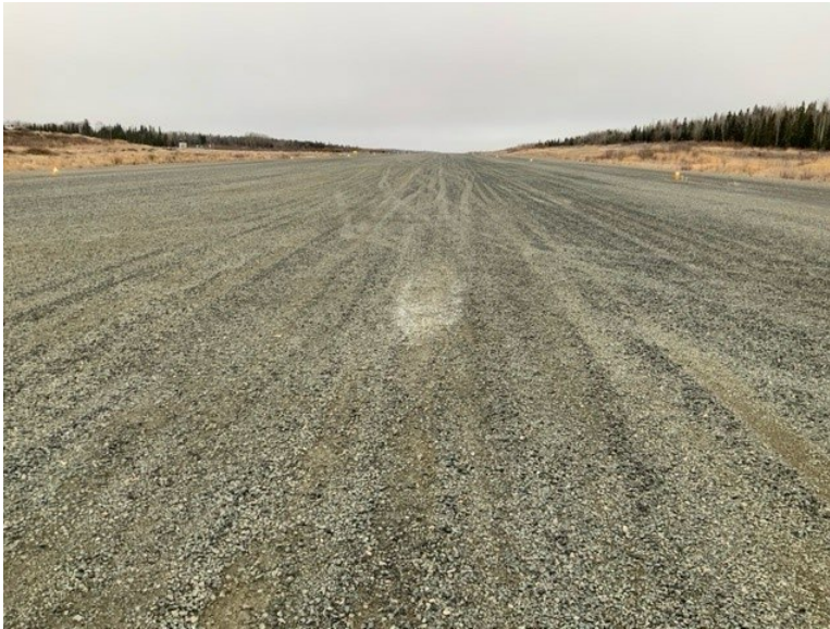
Figure 2. Impact mark made by aircraft's fuselage showing the touchdown point on Runway 29 (Source: Sandy Lake Airport)
