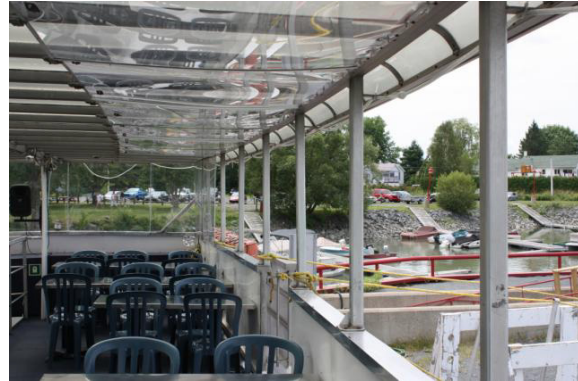
Photo 2. The upper deck hinged windows in raised position.
