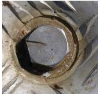
Photo 9. Typical hexagonal bolt on hatch cover
