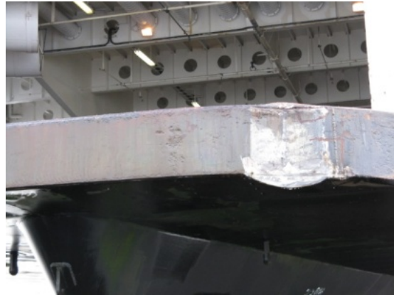
Photo 3. Damage to rubbing strake near centreline
