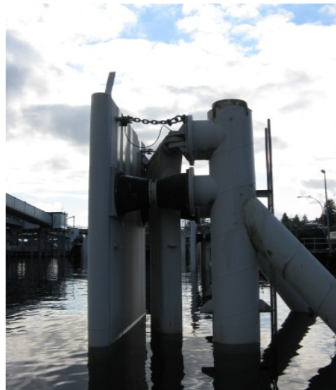
Photo 5. Undamaged starboard-side fender and articulated pad
