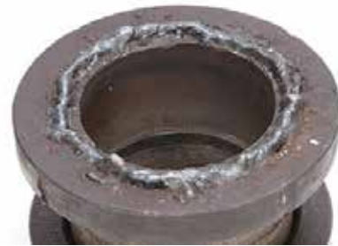
Photo 4. Weld repair on steel collar
