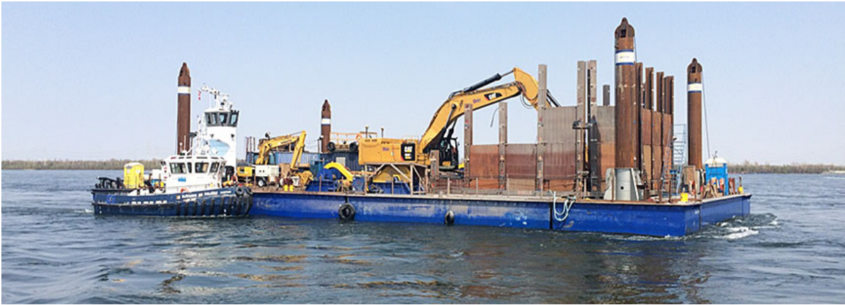
Figure 11. Barge with tugboats shown working at the sides (Source: Groupe Océan)
