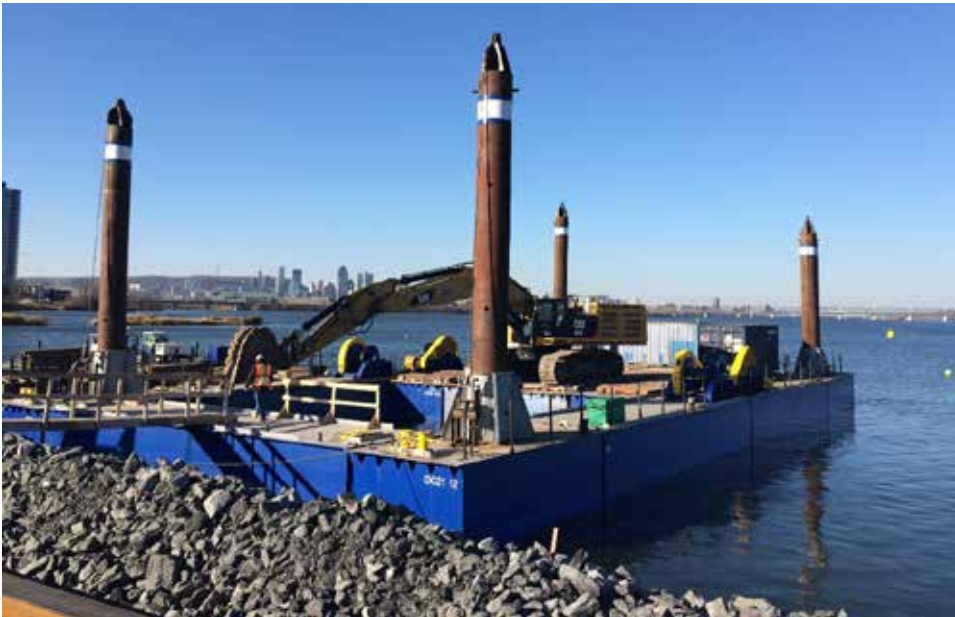
Figure 6. Excavation barge showing 4 spuds (Source: Groupe Océan)
