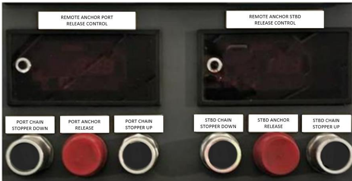
Figure 6. Remote release controls for the anchors (Source: BC Ferries, with TSB annotations)
