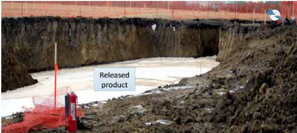
Figure 4. Existing excavation pit containing the released product
