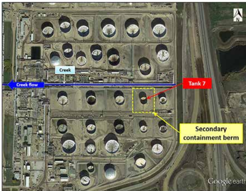
Figure 6. Tank 7 and its secondary containment berm (Source: Google Earth, with TSB annotations)
