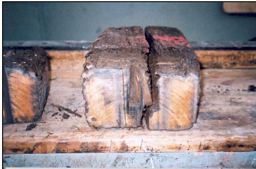
Photo 2. Defective tie condition, track G-5
