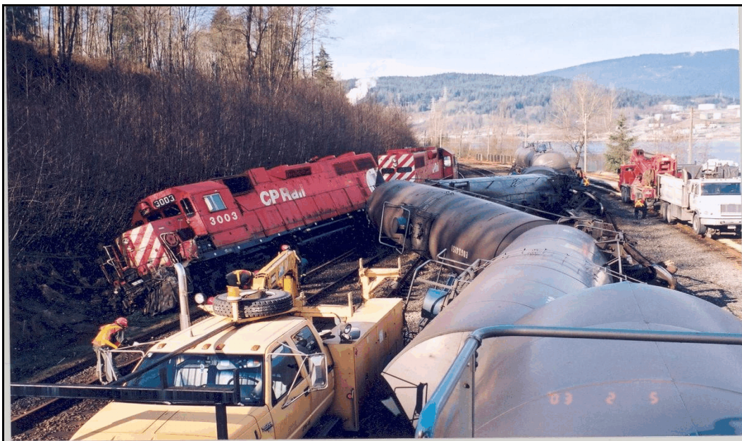
Photo 1. View of accident site
