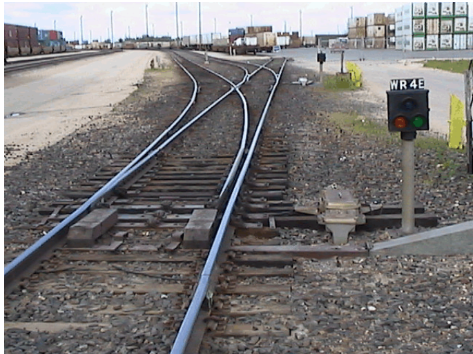
Photo 1. View looking westward into classification tracks at switch WR4E, Symington Yard (TSB photo) Switch aligned for movement into track WI03.
