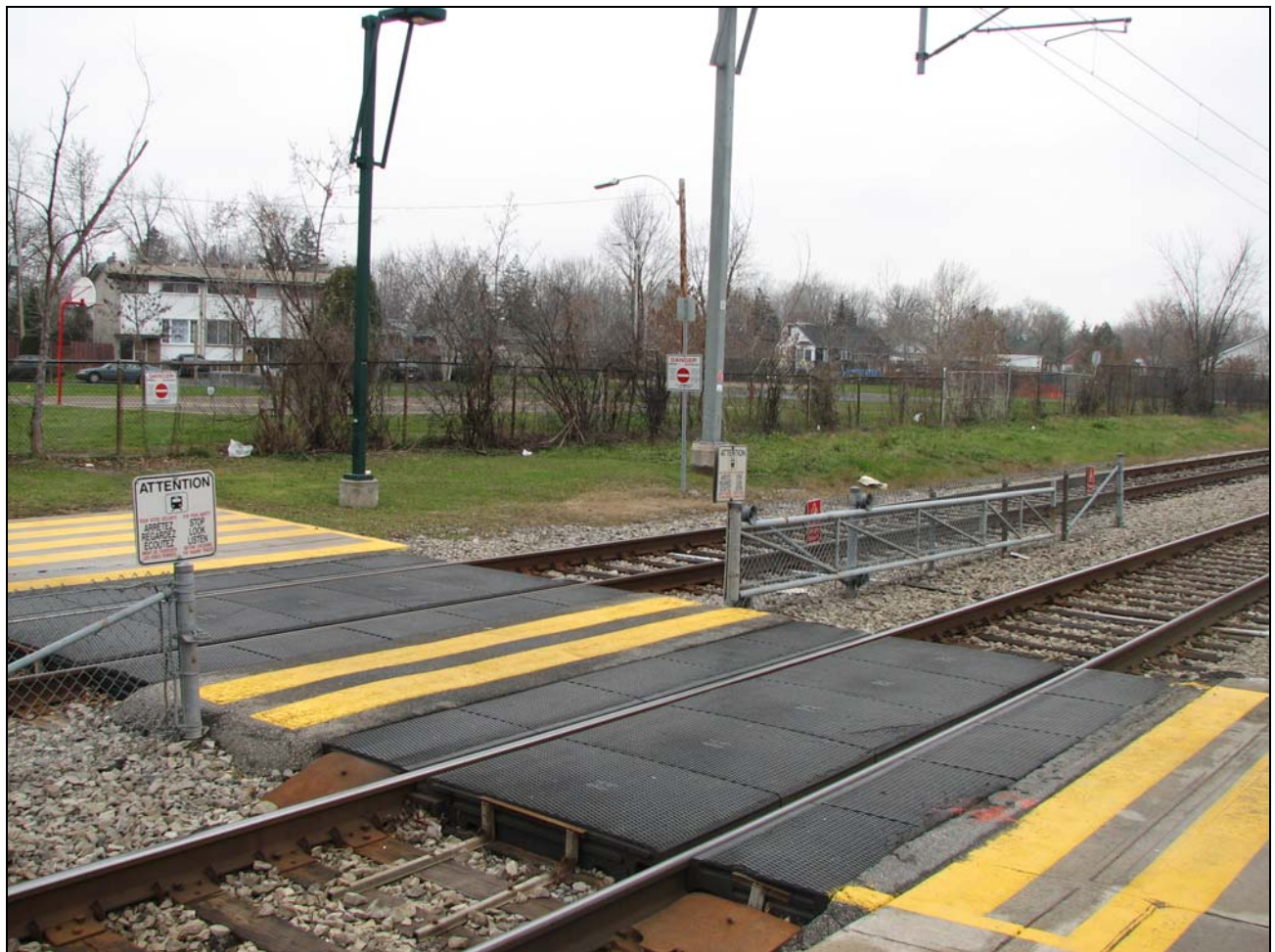
Photo 1. Platform link at the north end of the Roxboro-Pierrefonds Station
