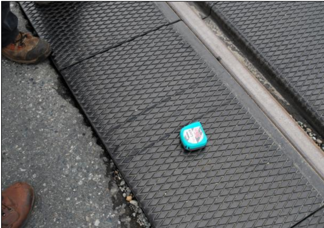
Photo 1. Tire marks on the west side of crossing
