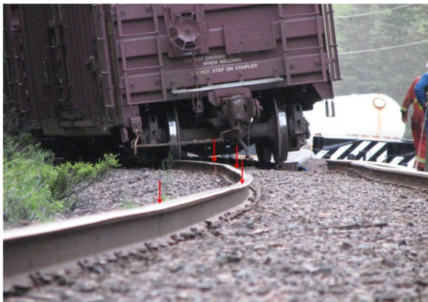
Photo 4. View towards POD. Arrows denote flattened rail condition.
