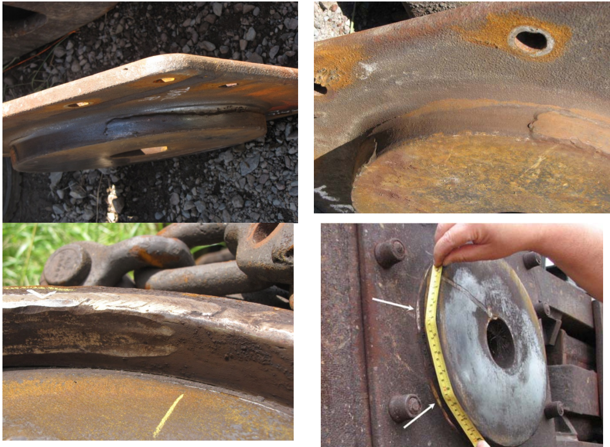
Photo 3. Center plate conditions on PROX 98433 - Built-up vertical surface with weld (top left and top right); Gouging in truck bowl wear ring at matching locations (bottom left); and shiny marks around base plate (arrows) from contact with truck bowl (bottom right).
