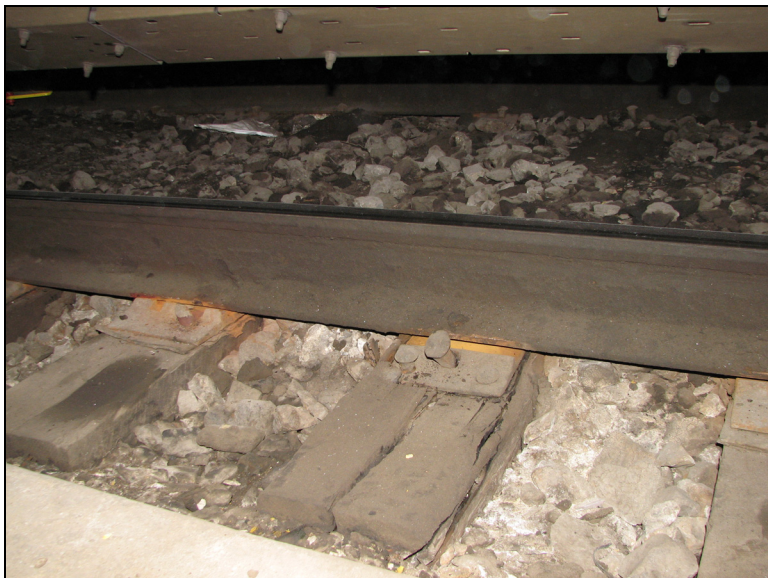
Photo 7. Ties, tie plates, track spikes and ballast
