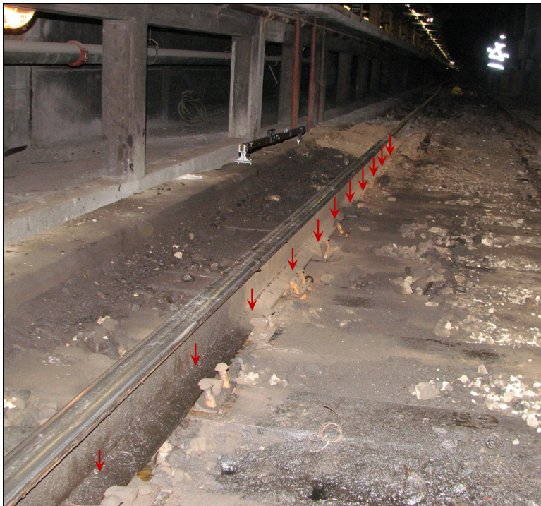
Photo 5. Locations of 10-inch tie plates with round spikes, indicated by red arrows – south rail
