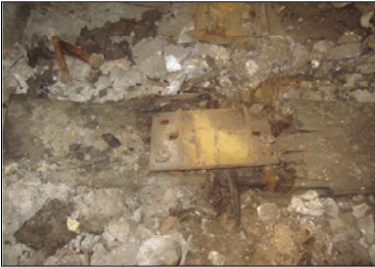
Photo 8. Closer view of tie, tie plate, track spikes and ballast
