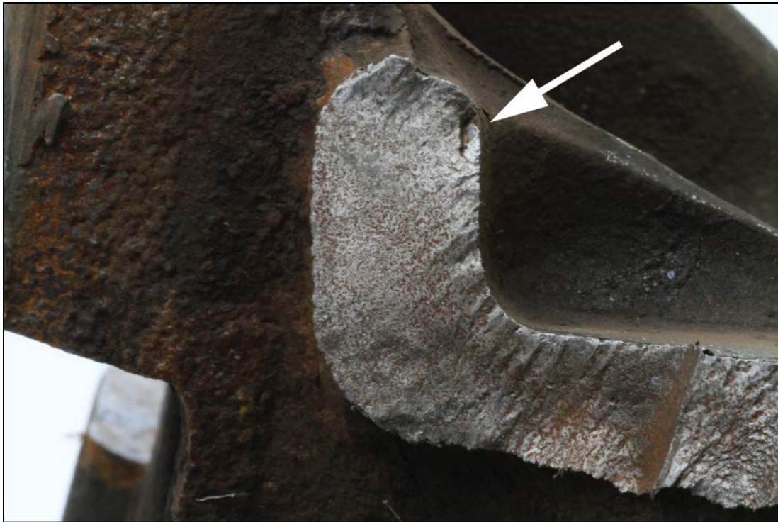
Photo 3. Close-up of origin area after cleaning (Note: The casting surface irregularity is visible towards the top right of the fracture surface.)
