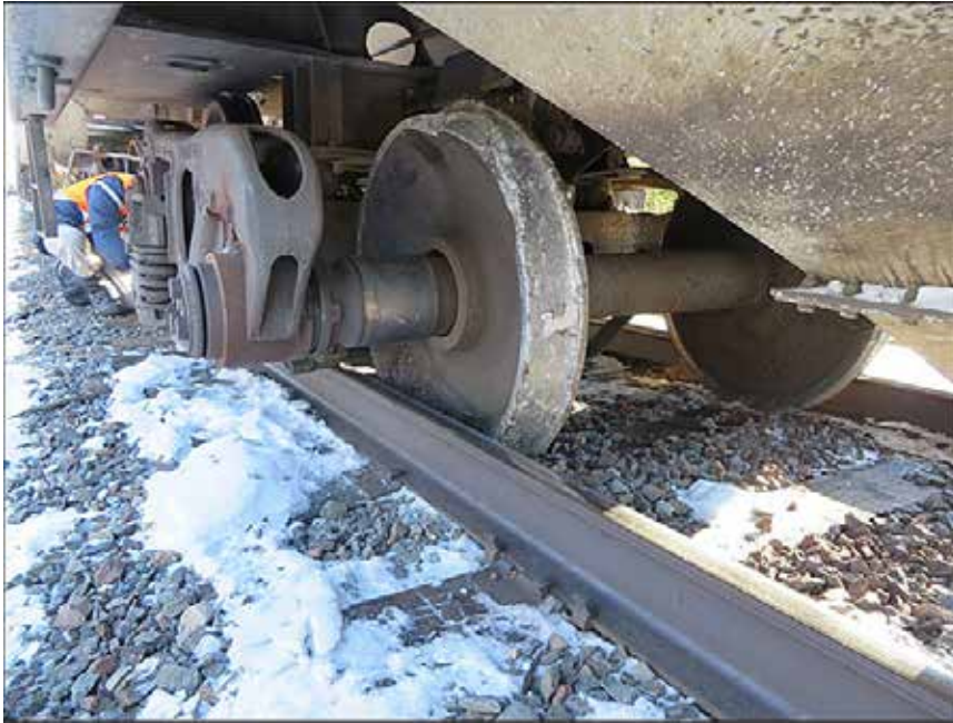
Photo 1. Derailed axle of car CRDX 15109
