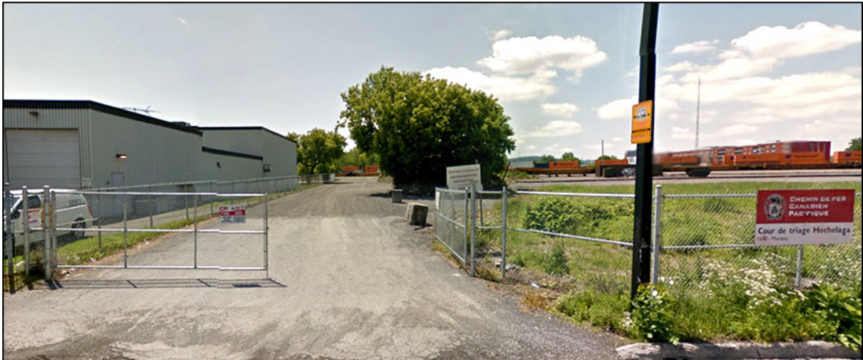
Photo 5. Chain-link fence in Hochelaga Yard (Source: Google Earth)
