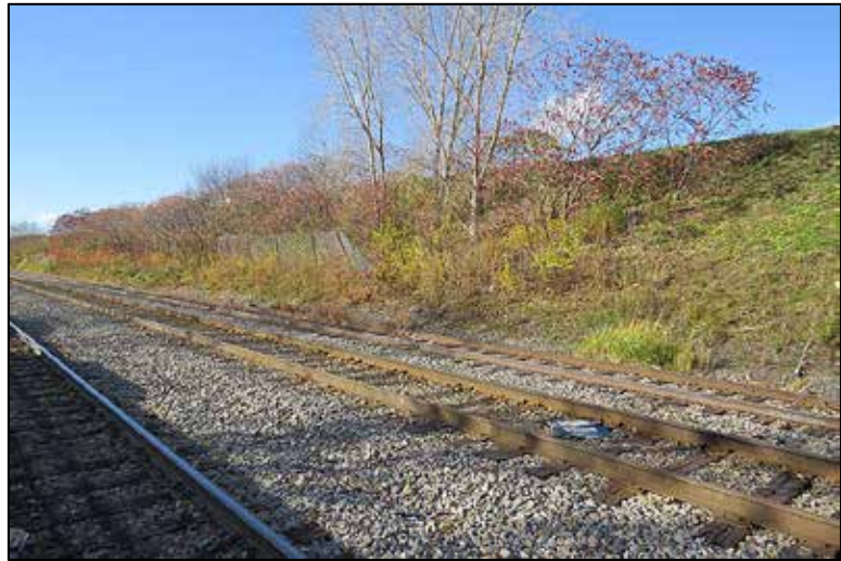
Photo 6. Poorly maintained or missing fence
