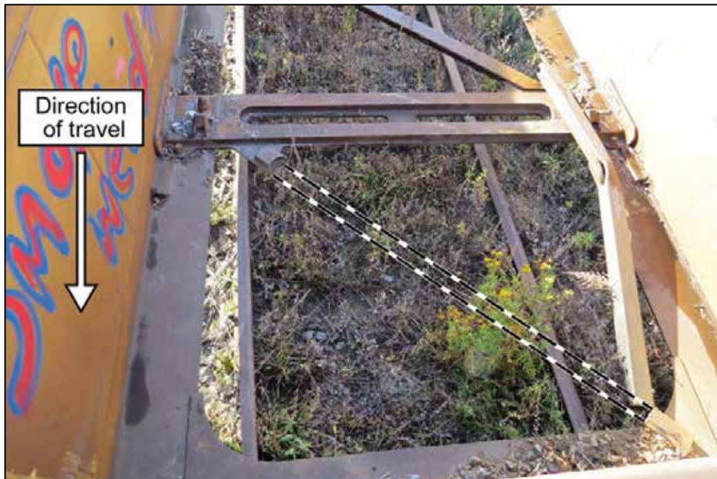
Photo 1. First diagonal member of the car decking (original position shown by dashed line)
