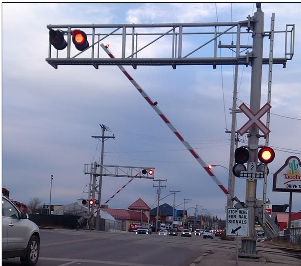
Figure 3. Photo showing the angle of the Central Avenue gates after the crossing protection had been activated for 10 seconds
