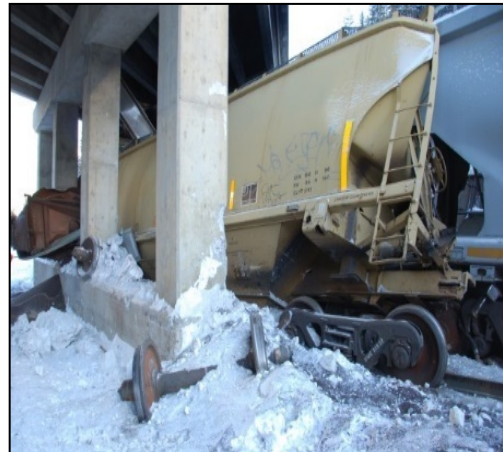
Figure 5. Cars under the Highway 1 overpass (Source: TSB)
