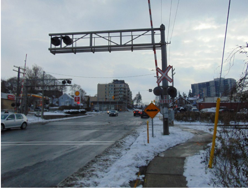
Figure 7. Lancaster Street West crossing, looking south (Source: TSB)
