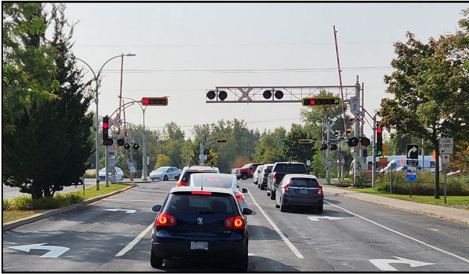
Figure 3. Intersection of Seigneurial Boulevard West and Route 116, looking south from Seigneurial Boulevard West (Source: TSB)
