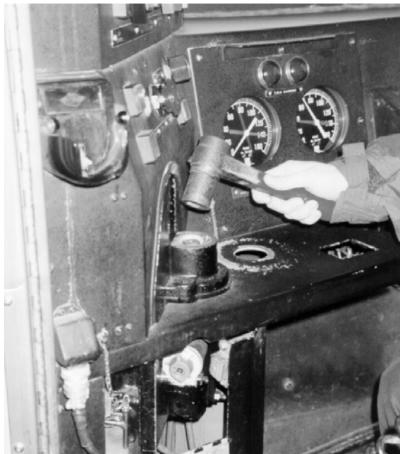
Figure 2 - Interior view of cab control station (automatic brake valve and handle storage location indicated by arrows)
